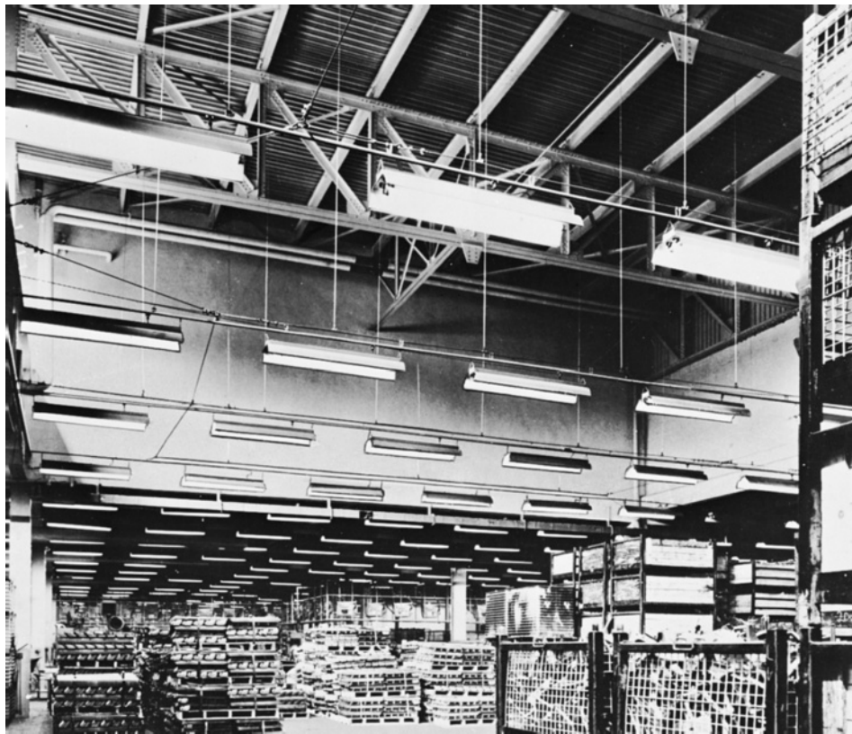
FIGURE 5-9 Typical trolley busway lighting system.
