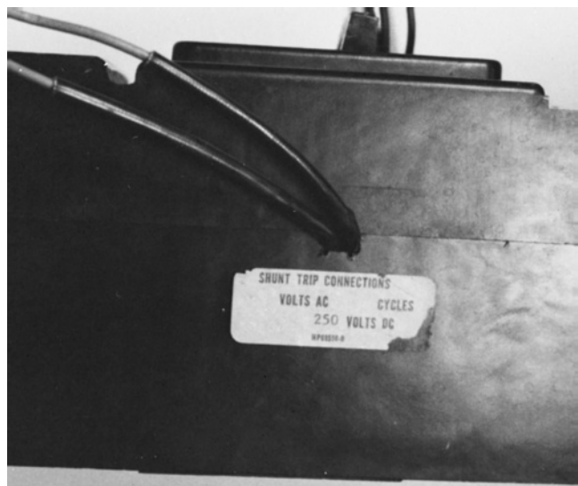
FIGURE 13-15 Shunt trip connection.
