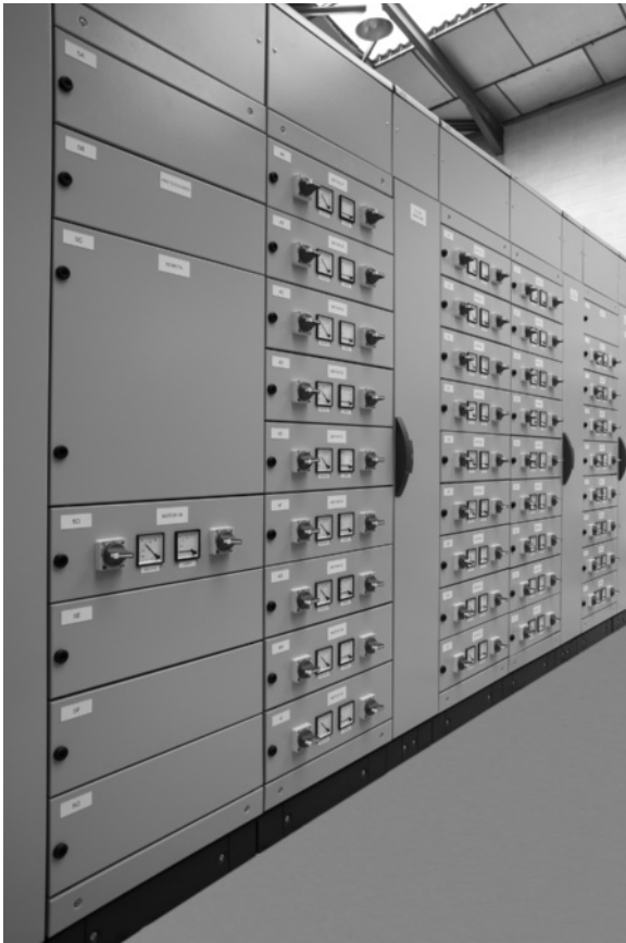
FIGURE 4-11 A typical power panelboard.
