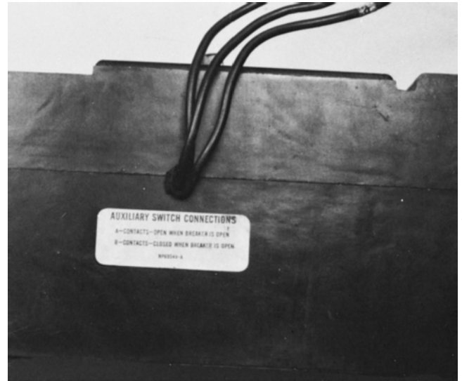
FIGURE 13-17 Auxiliary switch connection.
